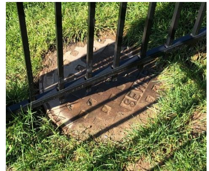
This fence illegally blocks City maintenance access to a sewer in a D&U Easement
