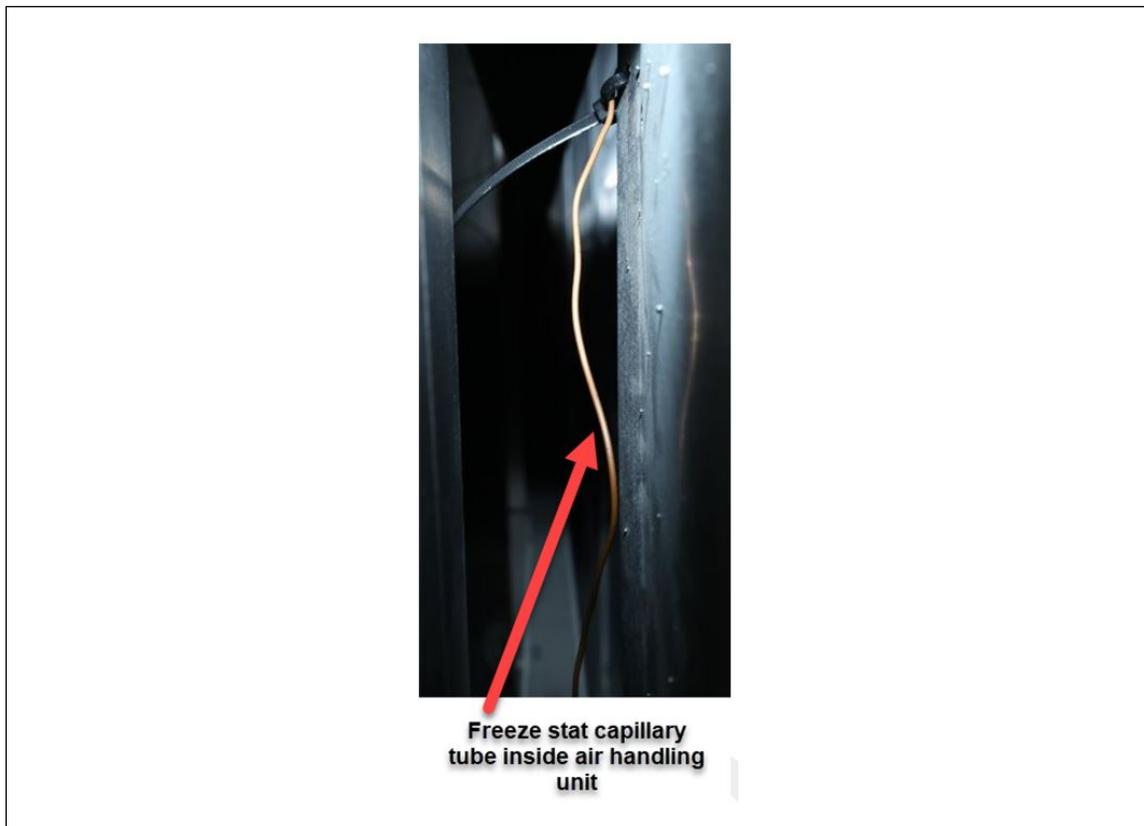
Fig. 3.5-4. Continuation of the freeze stat's copper capillary tube inside the air handler
