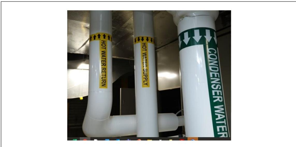
Fig. 3.5-2. Water lines for the heat transfer coils
