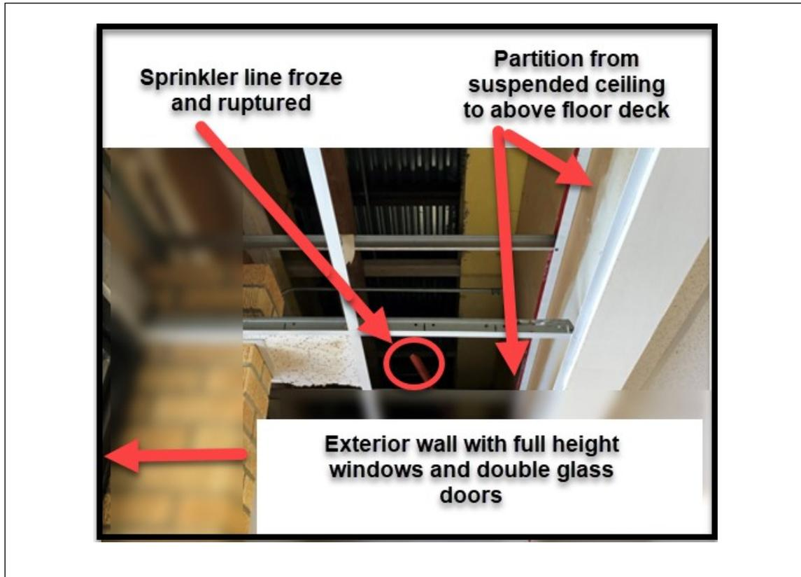
Fig. 3.4-1. Frozen/ruptured sprinkler line above suspended ceiling
